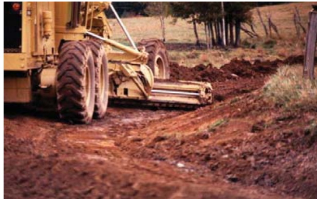
Ditching for Proper Drainage
